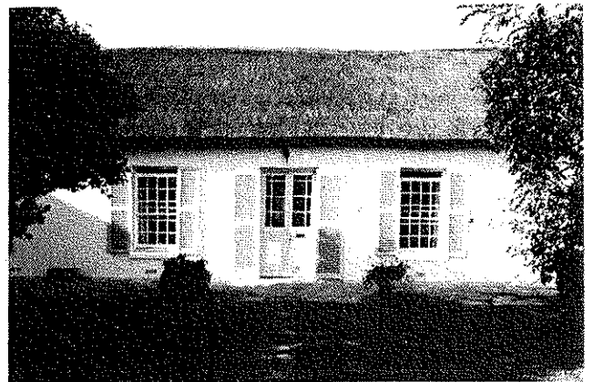
Fig. 11 Long Cottage, Durban Road
